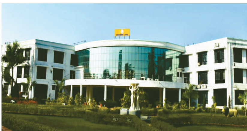
Administrative Building ANDUA&T, AYODHYA
