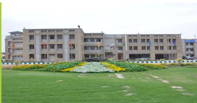
Administrative Building SDUA&T, MEERUT
