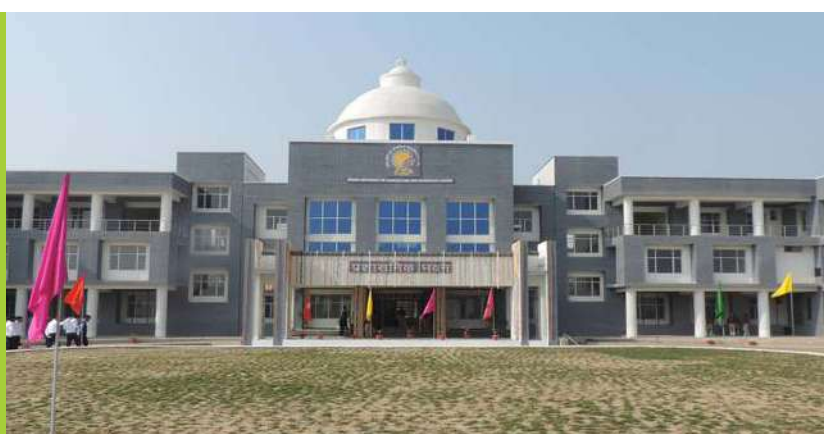
Administrative Building BUAT, BANDA
